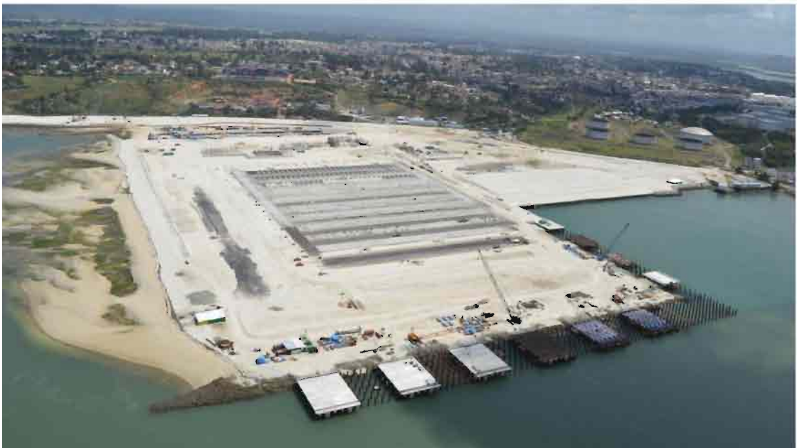
Figure 140. The proposed Lamu port under construction.
