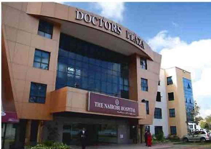
Figure 9. Nairobi hospital, Kenya is among the biggest hospitals in East Africa. (Built in April 1954)
