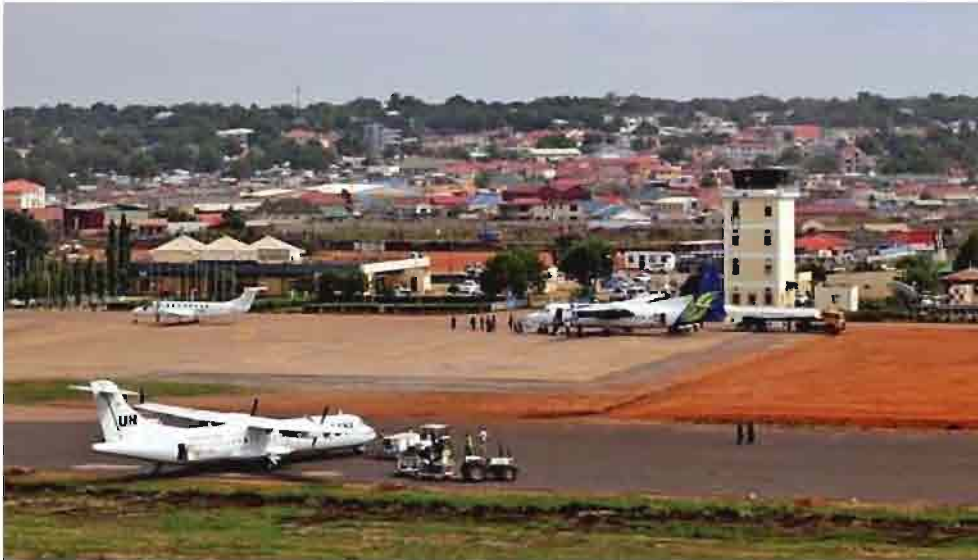
Figure 78. The Juba international airport.
