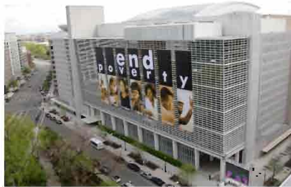
Figure 131. An example of a low oblique photograph of the World Bank headquarters (Washington DC, USA).
