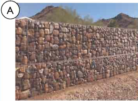
Building of check dams or gabions.
