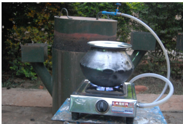
(B) Biogas plant.
