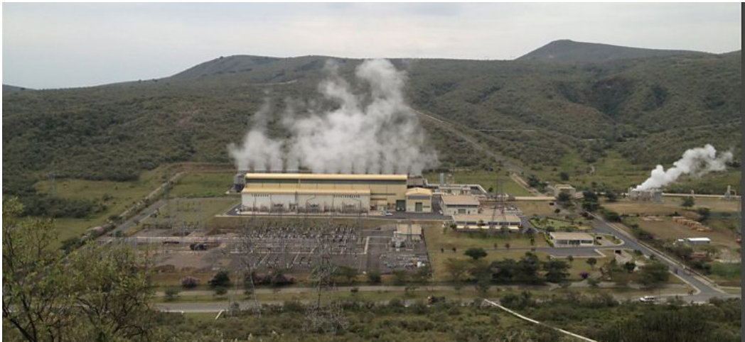
Fig. 5.16 Geothermal power station
