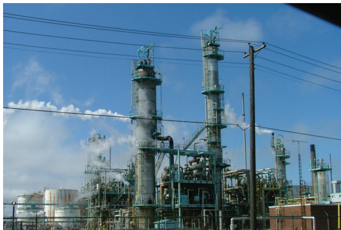
Fig 1.4 An Oil Refinery
