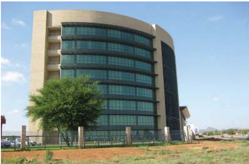
Gaborone, Botswana SADC headquarters building.
