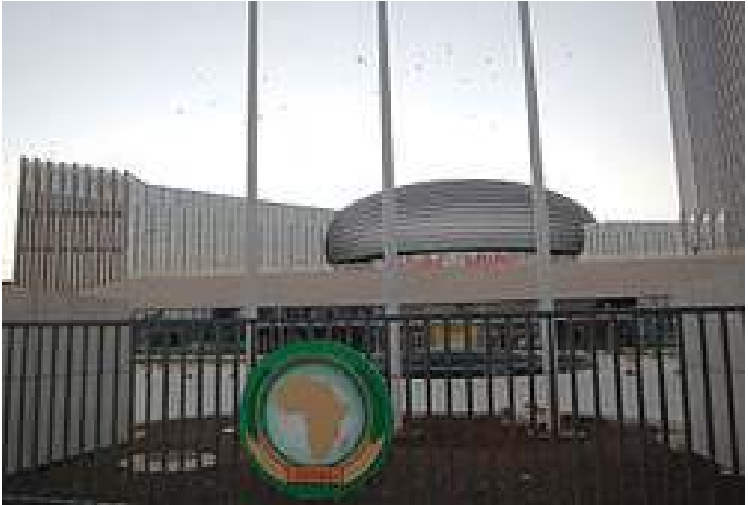
The AU headquarters complex in Addis Ababa, Ethiopia.
