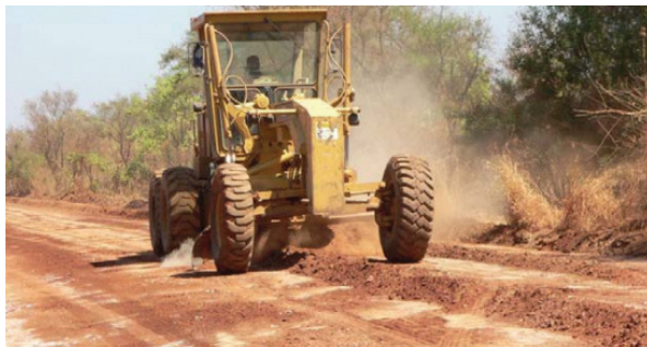
A road construction.
