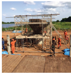
People building a bridge.
