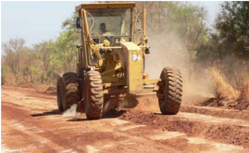
A road construction.
