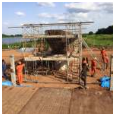
People building a bridge.
