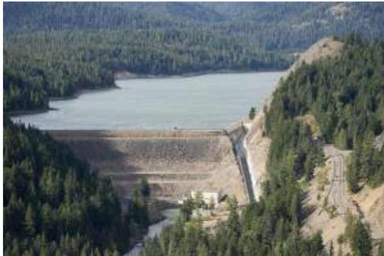
A dammed river.
