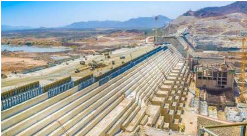
Figure 8.8 GERD (Grand Ethiopian Renaissance Dam) construction
