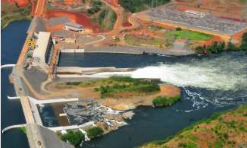
Figure 8.9 Bujagali Power Station in Uganda
