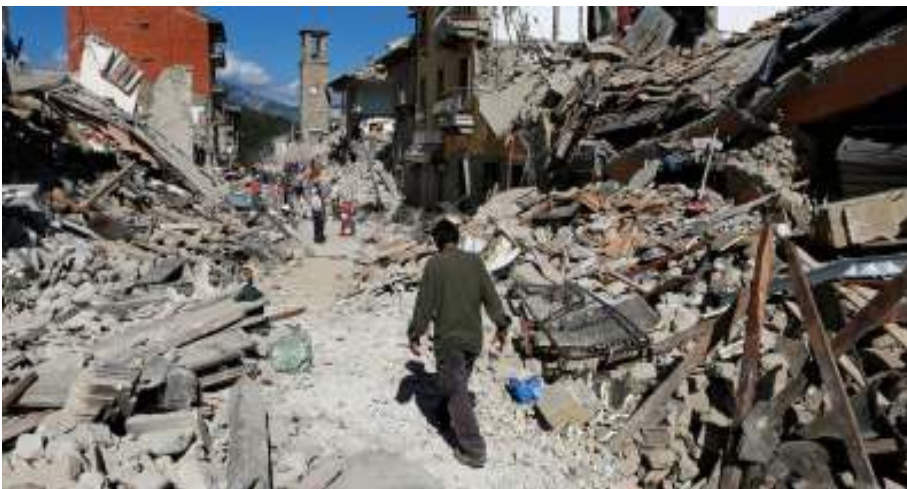
Figure 2.1 buildings destroyed by an Earthquake in Italy.
