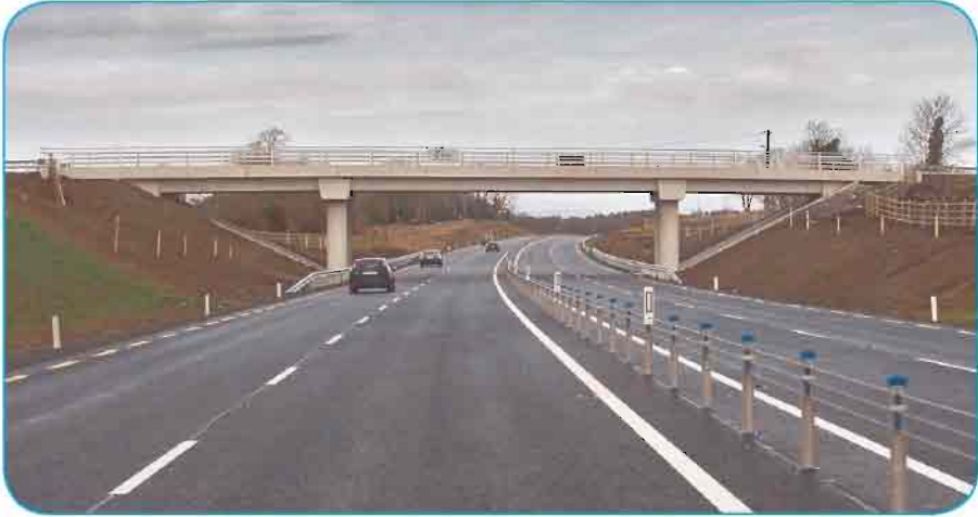
Construction of new roads.
