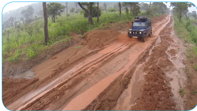
Poor road network.
