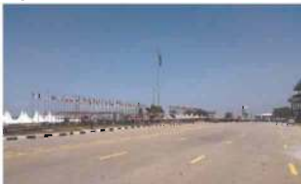
Construction of new roads
